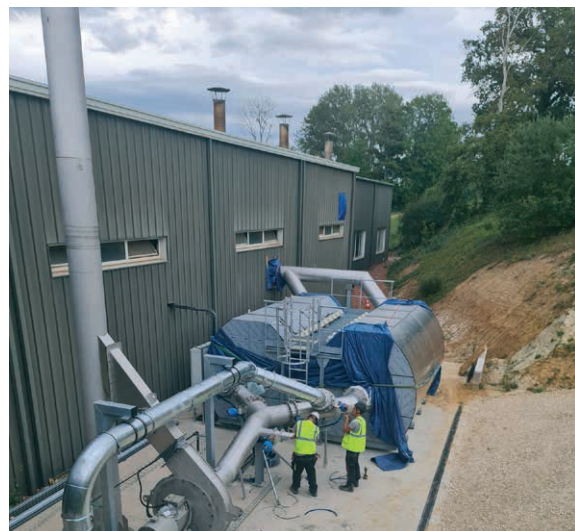
Installation of two Eco-Stocks® at the Pontigny site.
